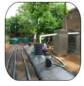
The Flexigester can be attached directly to a pour-flush toilet, capturing all the sewage. Removing the waste from the vicinity of the latrine can help to keep the latrine free from odours and flies, and encourage the use of the latrine over open defecation.
