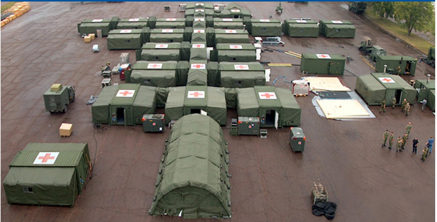
MECC™-based Field Hospital shelter system with ISO container linking corridors
