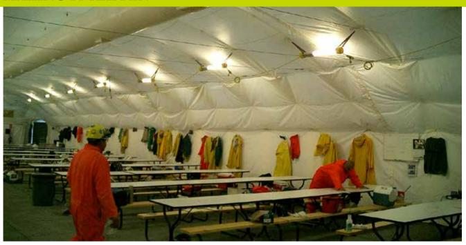
Blast resistant, lightweight, easy to customise and quick to deploy, Dynamic Air Shelters are unlike any other shelter solution in the world today. The system consists of a low-pressure air beam support structure, a heavy duty waterproof fabric shell and liner, and a flexible moveable exterior fabric barrier surrounding the perimeter of the shelter.
